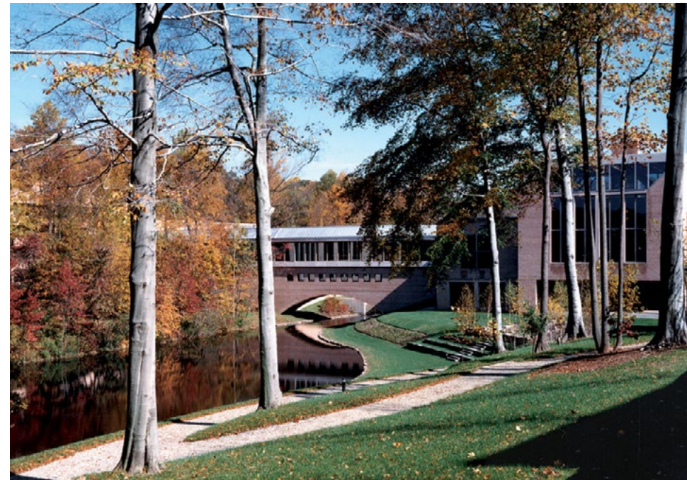
View east to the arched connecting bridge
