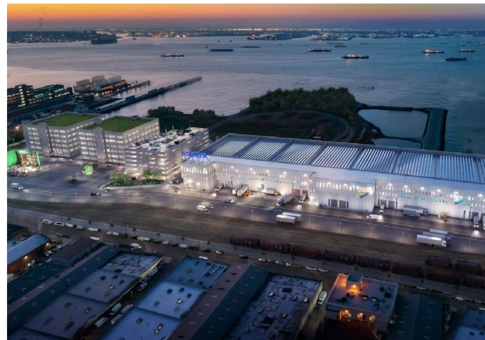
Steiner Studios Future Expansion at Bush Terminal
