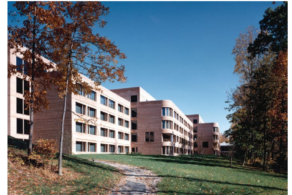
View of the north residential wing
