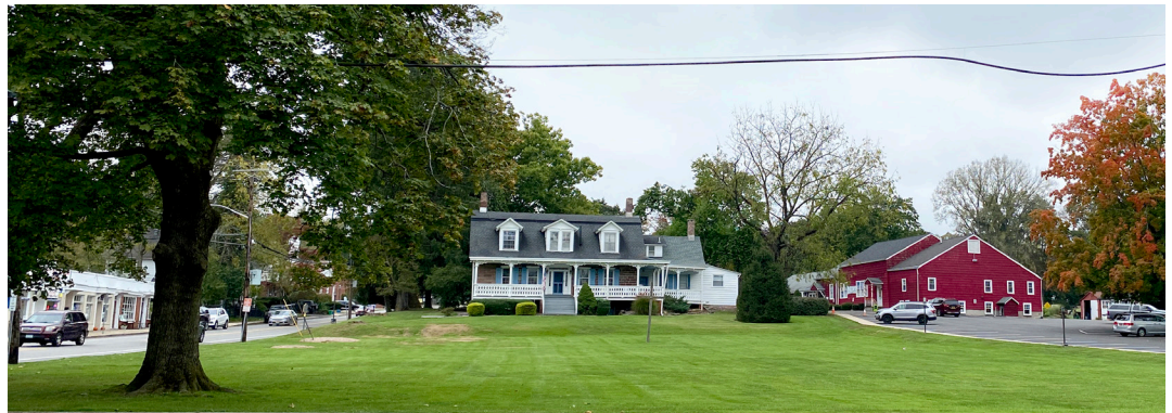
The Manse, home to Domine Samuel Verbruyck, Tappan © AKRF
