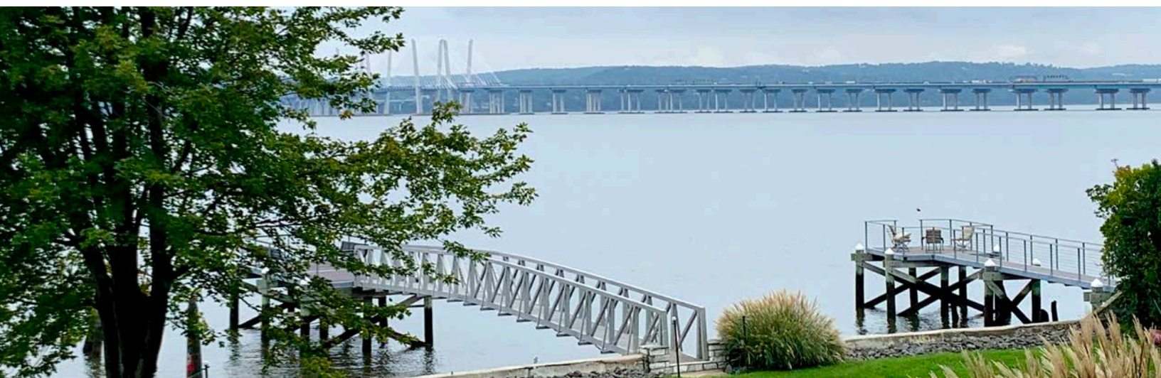
View of the Governor Mario M. Cuomo Bridge (Tappan Zee Bridge) from a private property © MUD Workshop
