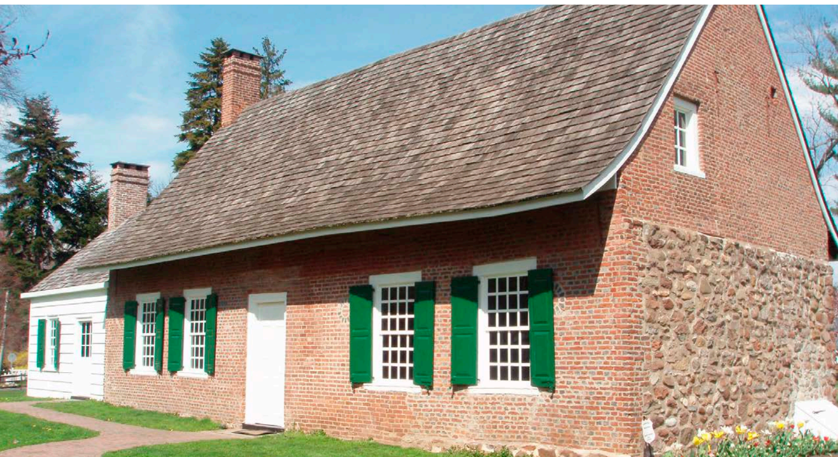
Dewint House, Tappan, built 1700. Source: WikiCommons
