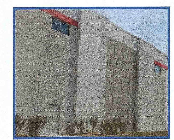
9 LAPPED PRECAST PANELS
