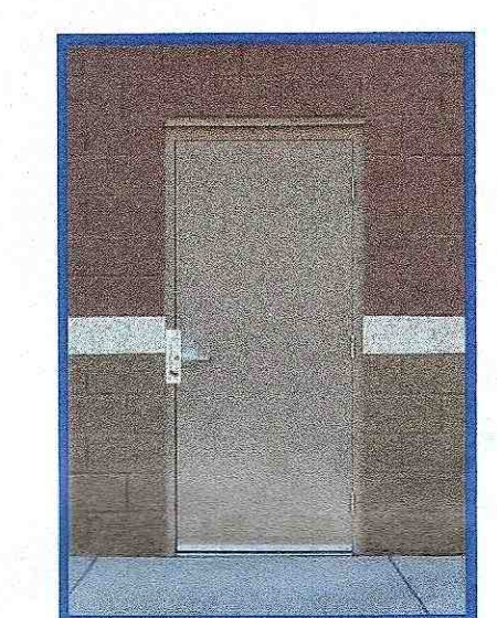
8 HOLLOW METAL DOOR & FRAME, PAINTED
