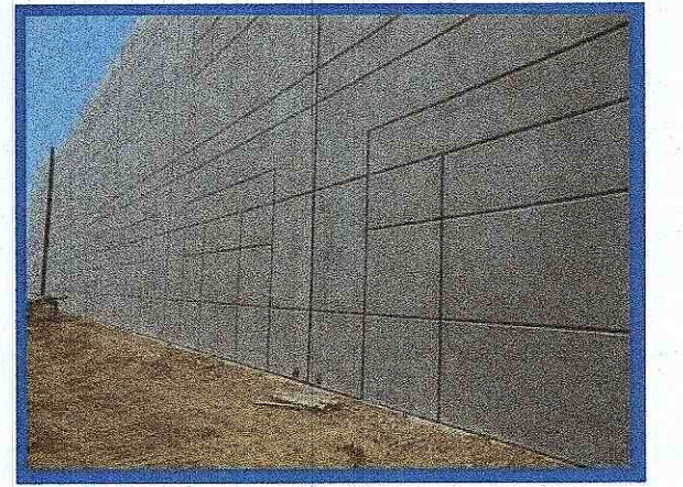
12 PRECAST REVEALS (HORIZONTAL & VERTICAL)
