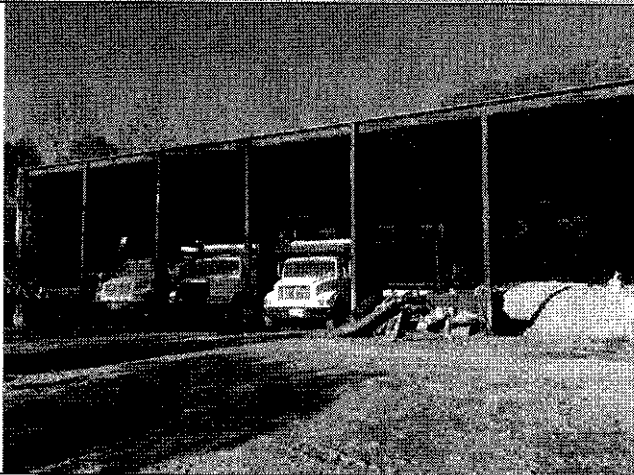
Description: Standing along southern property line, looking north at existing building.
