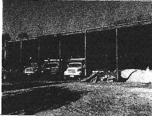
Description: Standing along southern property line, looking north at existing building.
